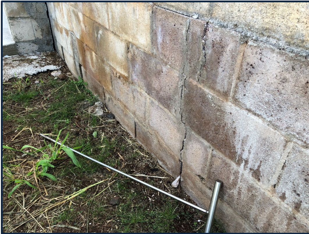
Photo No. 13 (November 12, 2020) – Additional cracks on same CMU retaining wall as previous picture. View of north side of retaining wall looking northeast.
