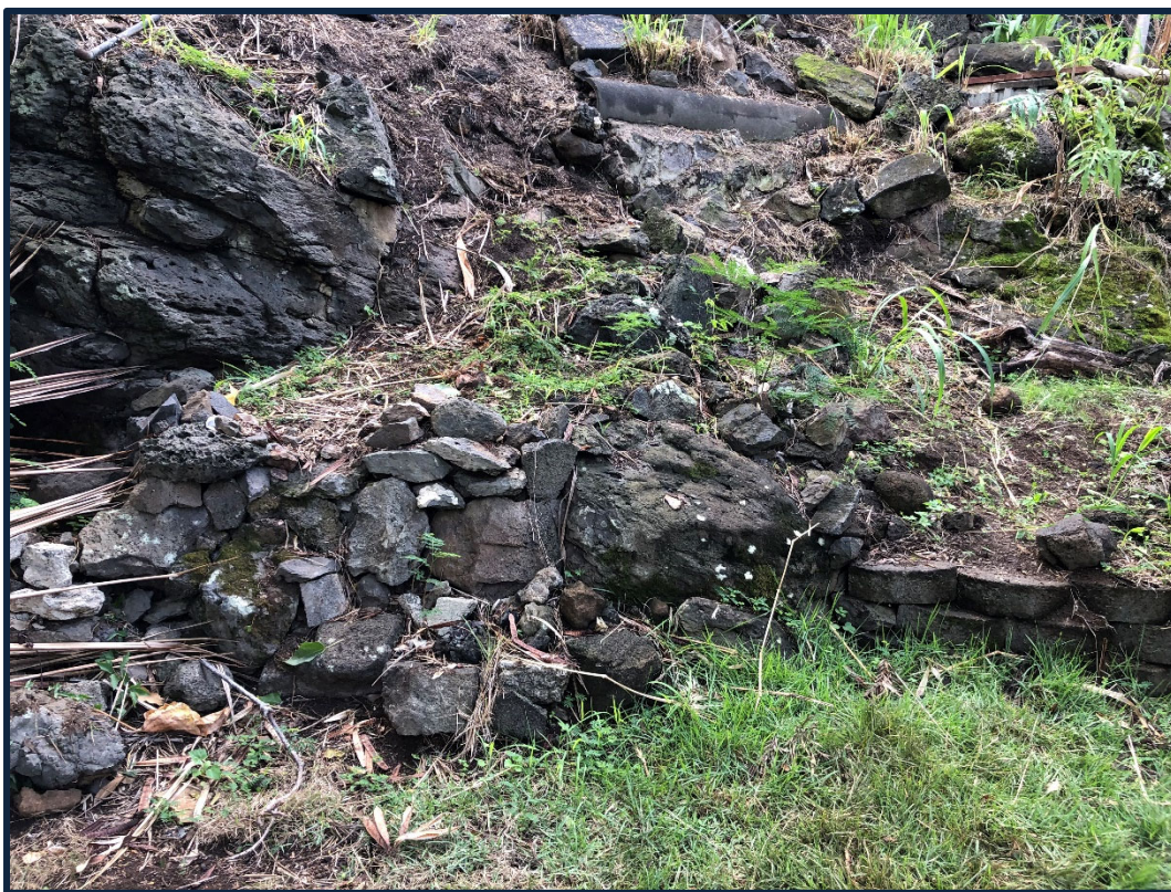
Photo No. 11 (November 12, 2020) –Eastern and central portion of slope. Note the manmade dry stack wall constructed near the base of slope.
