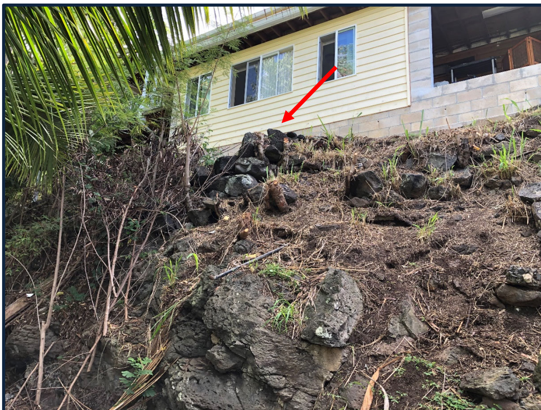
Photo No. 9 (November 12, 2020) – East side of slope. Note the loose pile of boulders stacked near the top of slope. .
