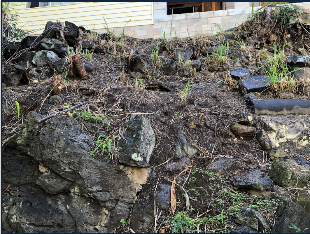
Photo No. 8 (November 12, 2020) – Eastern half of slope. Note the loose soil and rock material in the central portion of the slope near the abandoned pipe.
