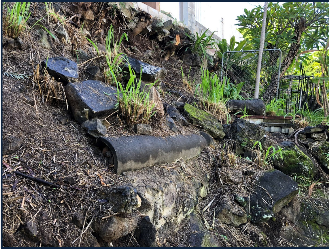
Photo No. 7 (November 12, 2020) – Central portion of slope where the abandoned concrete pipe was discovered during the previous reconnaissance. Pipe supported by grouted CRM.
