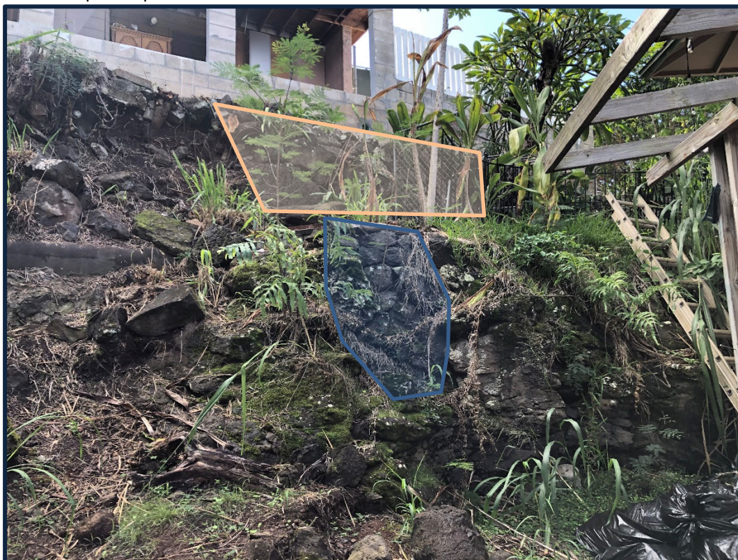
Photo No. 10 (November 12, 2020) – West side of slope. Note the section of dry stack cobbles used to extend the natural rock formation ledge (blue highlighted section). The upper “retaining wall” also consists of dry stack cobbles and boulders (orange highlighted section).
