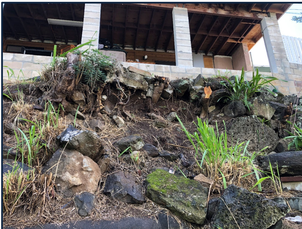
Photo No. 6 (November 12, 2020) – West side of slope. At the top of the slope, an undermined “lip” of grouted rubble (including cobbles and concrete blocks) was observed.
