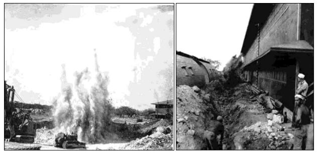
Figure 17. Photographs of blasting for pool construction north of the Seabee Camp (left) and for underground utilities at MCAS Ewa (right) (source: 130<sup>th</sup> NCB 1945).
