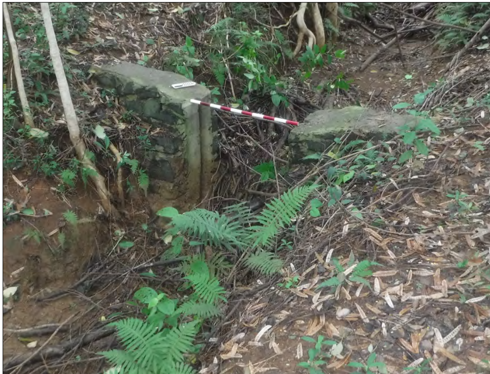
Figure 26. Feature 7 (Site 1), dressed basalt block and mortar sluice gate, view northwest
