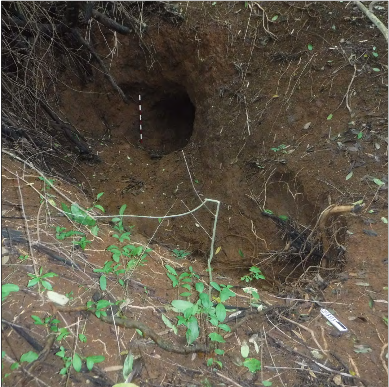
Figure 40. Hand-excavated culvert through dense clay (Feature 1 at Site 8) under historic dirt road; view northeast
