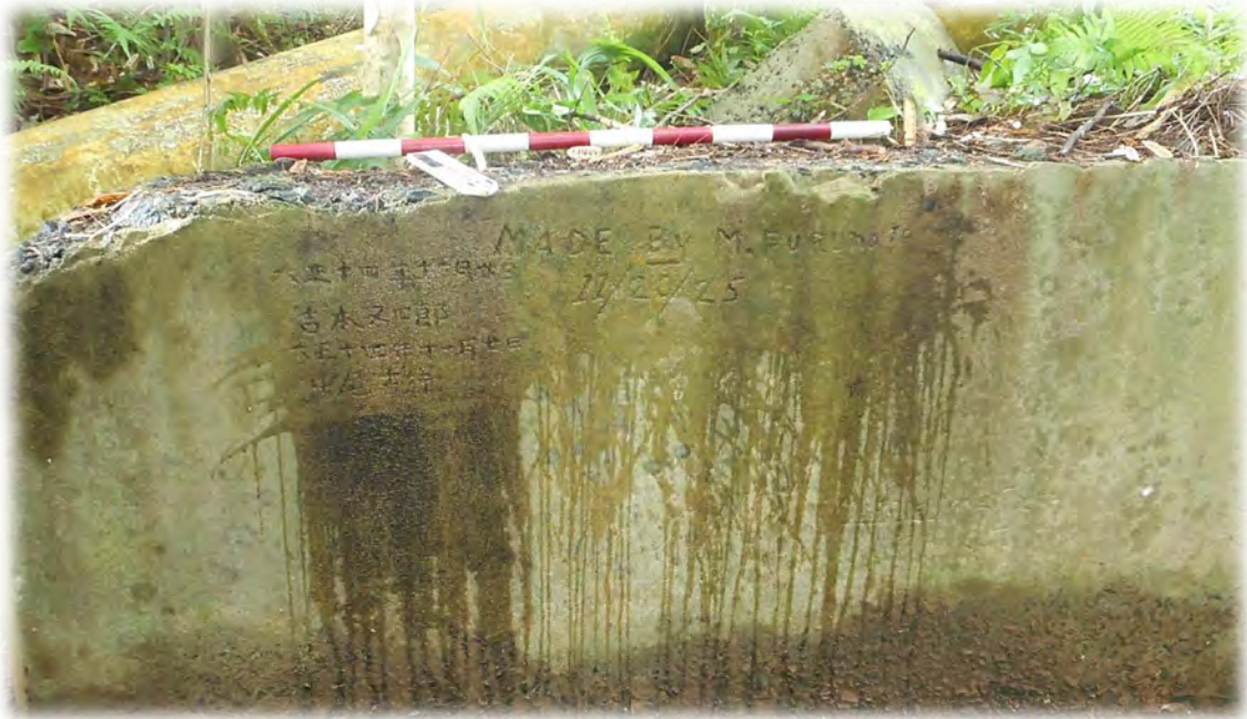
Detail of concrete irrigation-ditch feature with inscriptions from its builders in 1925
