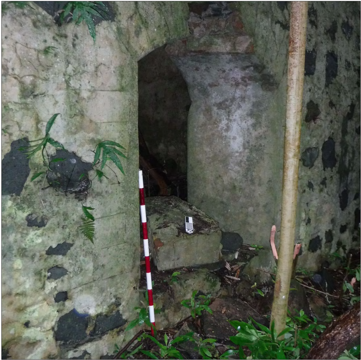
Figure 35. Doorway to pump house structure (Feature 1 at Site 5), view south
