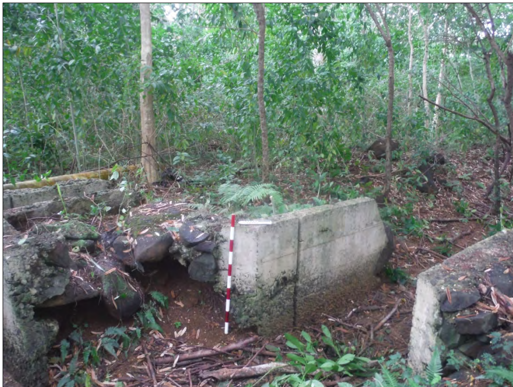
Figure 15. Overview of Feature 2 (Site 1), view east; note, natural boulders incorporated into concrete construction.
