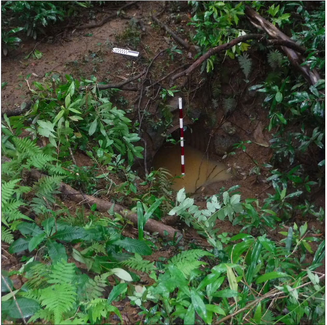
Figure 38. Detail of culvert at Site 6, view east
