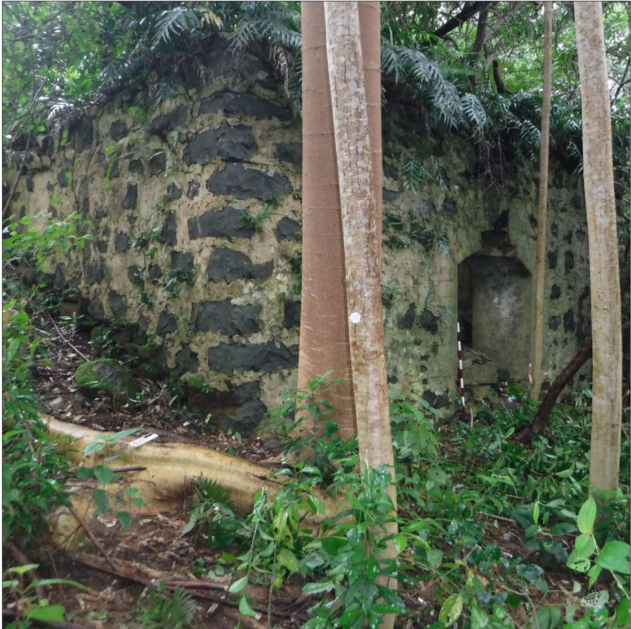
Figure 34. Pump house structure (Feature 1 at Site 5), view southeast
