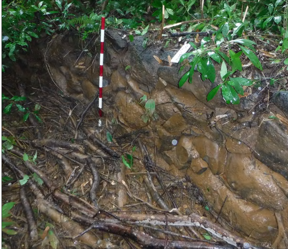
Figure 25. Feature 5 (Site 1), representative section of well-constructed (dry-stacked) boulder irrigation ditch wall
