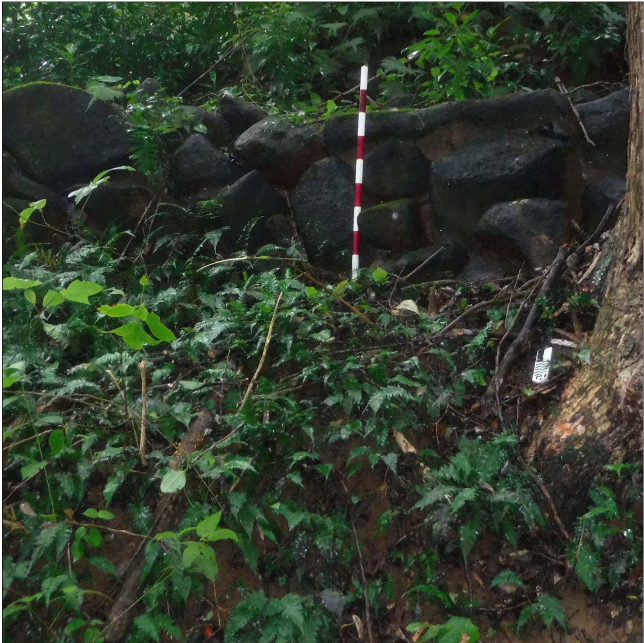
Figure 39. Central portion (detail) of dry-stacked retaining wall, view south
