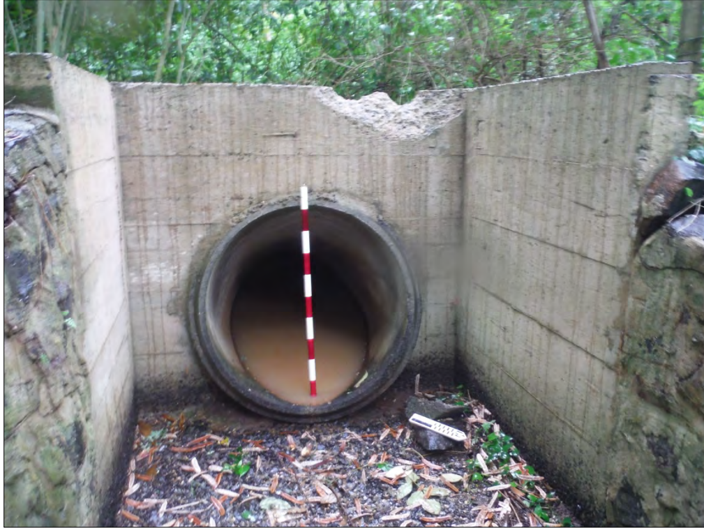
Figure 21. Culvert portion of Feature 3 (Site 1), view southwest.
