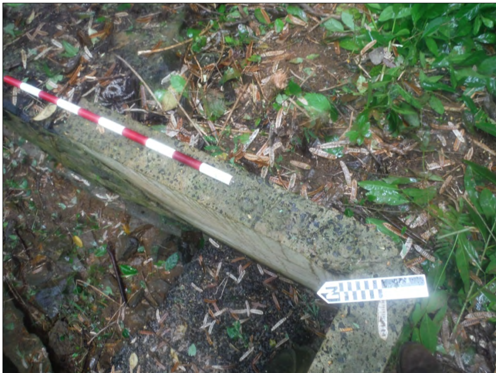
Figure 22. Inscription on poured-in-place concrete portion of Feature 3 (Site 1), reading "6/3/60."
