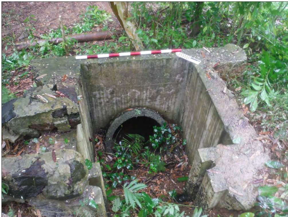
Figure 23. Portion of Feature 4 (Site 1), view northeast; note, sluice gate grooves in lower portion of image
