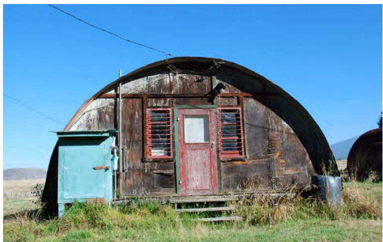
Quonset Hut Dormitories - Photo: Ho'okuleana LLC
